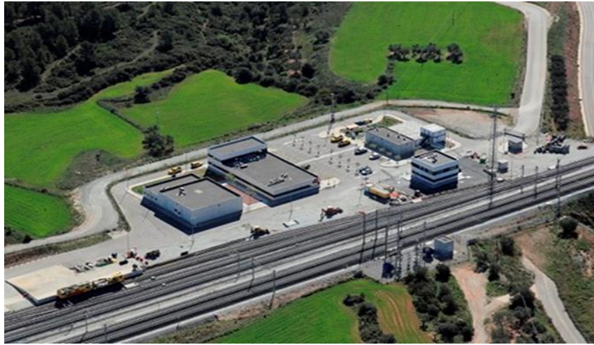
Figure 5 - LFP maintenance site for railways tests and trials
