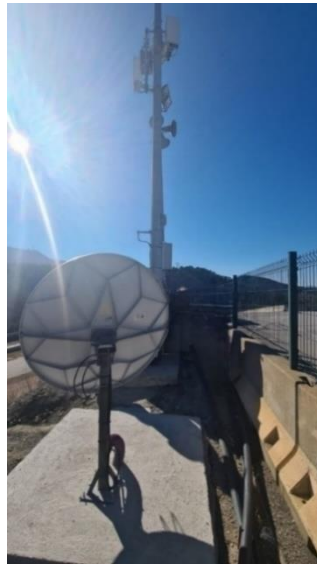
Figure 55: VSAT deployed in the circuit of Castellolí
